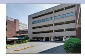
This 6-level garage serves visitor, physician, and patient parking at the largest ambulatory care center in the Northeast. It is a precast concrete structure with double tee floor slabs, architectural precast wall panels with a smooth aggregate finish, and two hydraulic passenger elevators. It is connected directly to the Medical Plaza Building on each or its four lower levels. A pedestrian bridge provides direct access to the acute care facilities at Hackensack University Medical Center.
