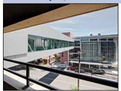
The Medical Center has four major pedestrian bridges, two of which span public roadways connecting the John Theurer Cancer Center and its associated garages to the main hospital complex. The bridges, which are of steel truss construction clad in aluminum and glass, are fully climate controlled and vary in length from approximately 100 to 300 feet.
