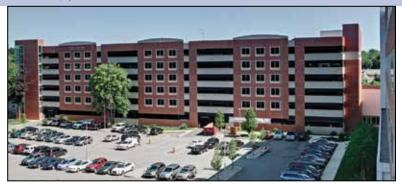
This 5-level parking garage at the Morristown Medical Center is a galvanized steel frame with "Filigree" concrete decks. The exterior of this garage is clad with precast concrete and thin brick panels. The interior is fully sprinklered and has two high speed "machine roomless" traction elevators and three stair towers. It was constructed in two phases and now totals approximately 1300 spaces.
