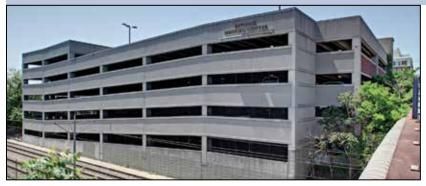
This 5-level garage is located on Avenue E in Bayonne adjacent to the hospital campus. The precast concrete structure, with double-tee floor construction and stairway/elevator towers at either end, features perimeter spandrels with brick infills.
